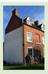
Thickness not 220mm but 345mm -- a brick and a half -- Insulated with 40mm woodfibre - 8mm lime plaster -- without a VCL
